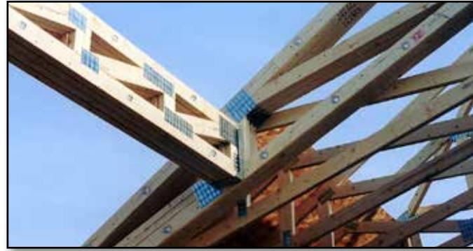
**⚠ WARNING!** All of the plies in a Truss Girder must be fastened together completely in accordance with the requirements specified in the TDD **before** attaching any supported members or other loads to the girder.
