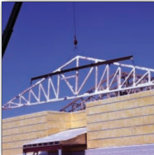
Erecting the trusses on the jobsite
