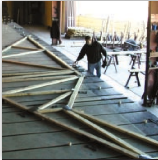
Manufacturing the trusses
