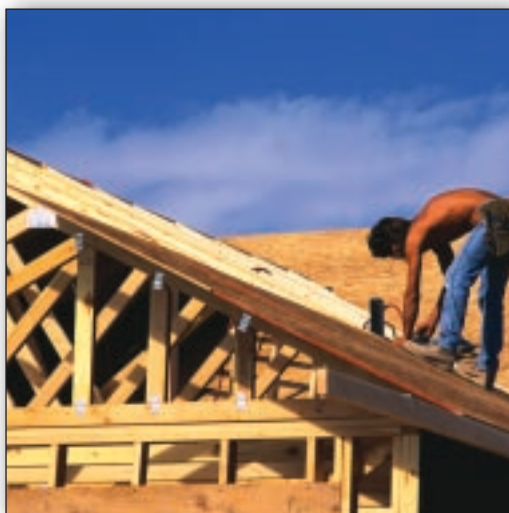
Permanent bracing system
